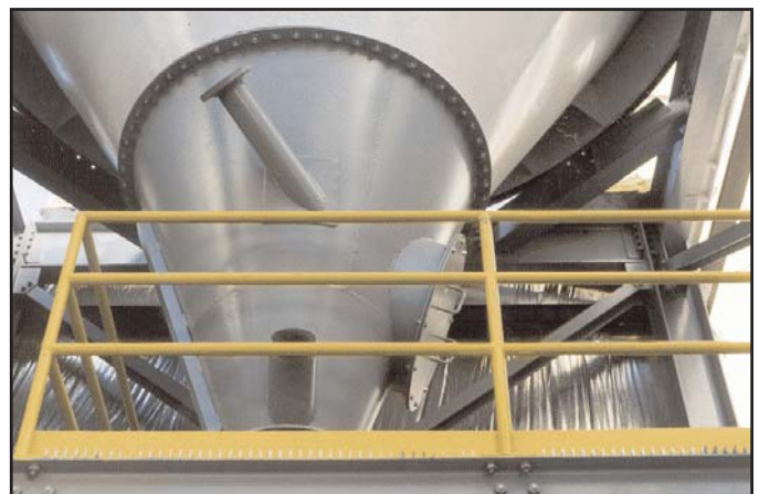
70 degree secondary hopper to improve dust discharge.
