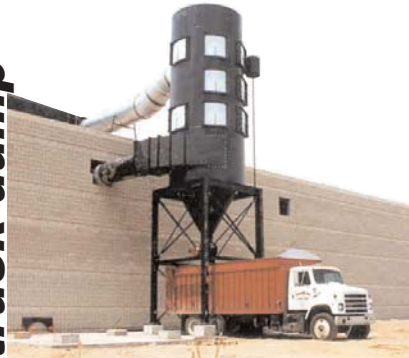
The 276AC10 filters can be mounted for truck dumping.
